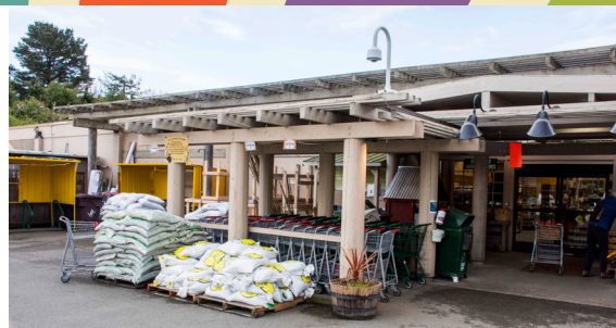
The north entrance cedar trellis
